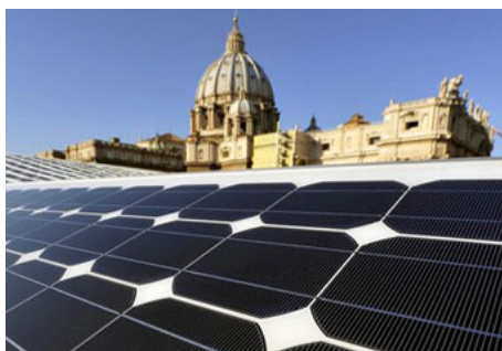
Solar electric panels atop the Vatican in Rome
